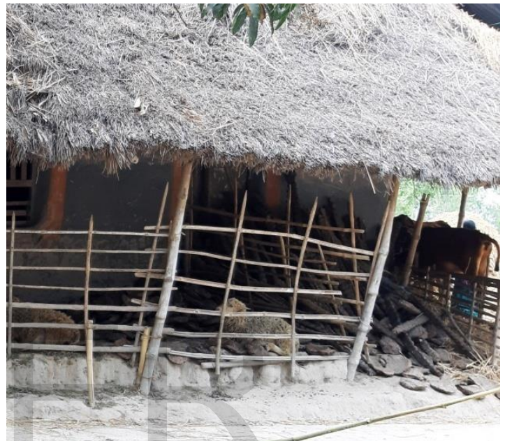
Fig5: Roofing material of the houses.
