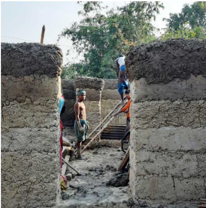
Fig6: Thick mud is used for erecting the wall
