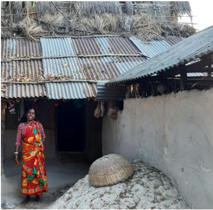
Fig12: Tin sheets are used for roofing
